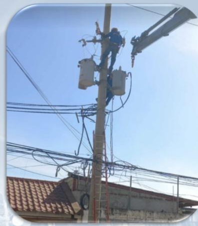
Various projects for the replacement of distribution transformers
